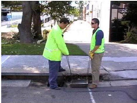
Plate 13 Lift grate and move grate to one side
