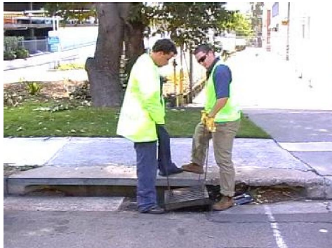
Plate 14 Lift grate above the support frame
