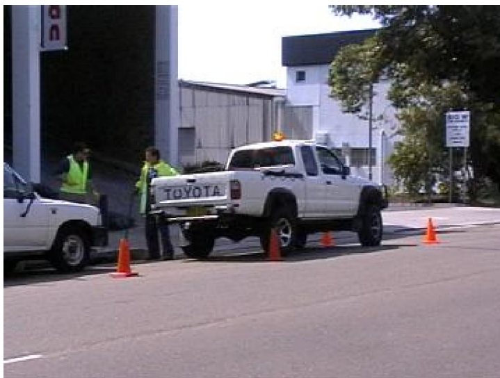
Plate 1 Vehicle positioned near pit, preventing traffic from passing close to the pit.
