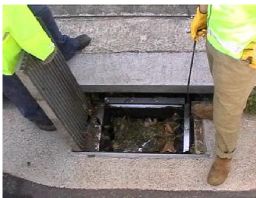
Plate 18 Lift the bag from the cage and support frame
