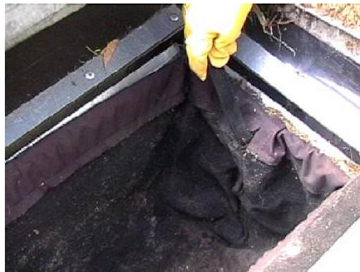
Plate 26 Ensure that the unit is positioned correctly, with the lifting loops on the inside
