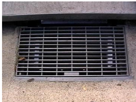
Plate 28 Installed filter bag and sealed pit
