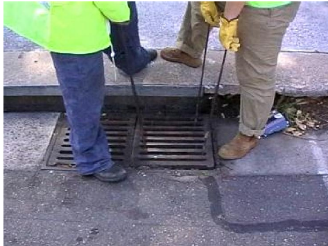
Plate 12 Position each lifter either side of the grate
