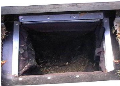
Plate 27 Correctly installed filter bag
