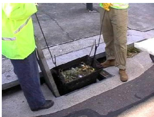
Plate 19 Lift the bag from the stormwater pit
