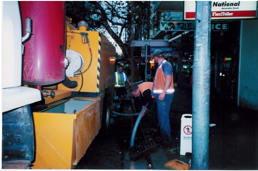
Plate 16 Cleaning an Enviropod using the inductor method
