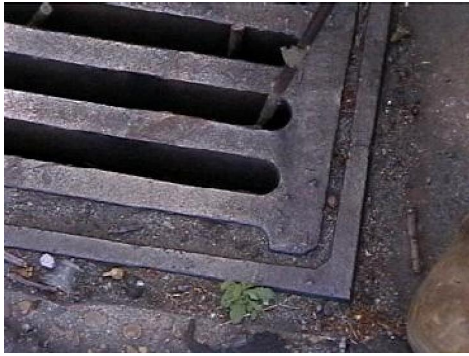
Plate 11 Insert hook near edge of grate
