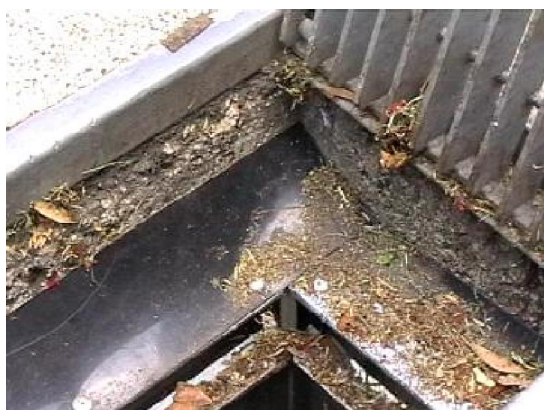
Plate 29 Check seals are pushed against the pit walls
